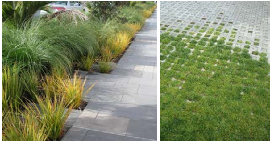
Figure 69. High quality unit paver integrated with WSUD in local centre (Source: Design Flow)
